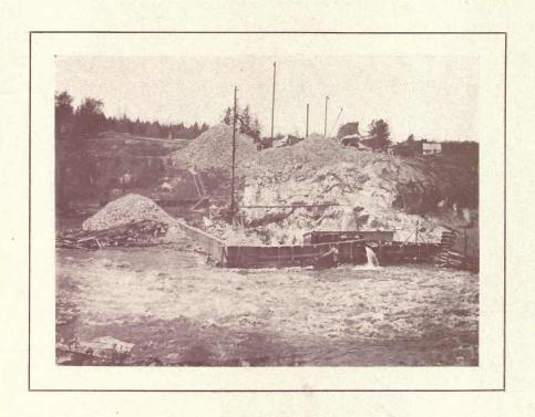
ERE is shown the condition of the work on June ninth. On this day the excavation for the power house being complete and the preparations of the foundations for the dam being in order, concreting was begun.
